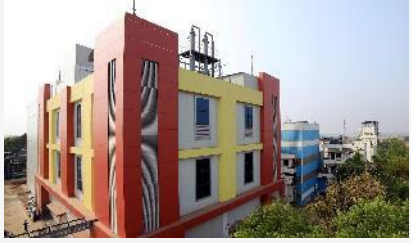
Additional Clean Room Facility, Bidar
